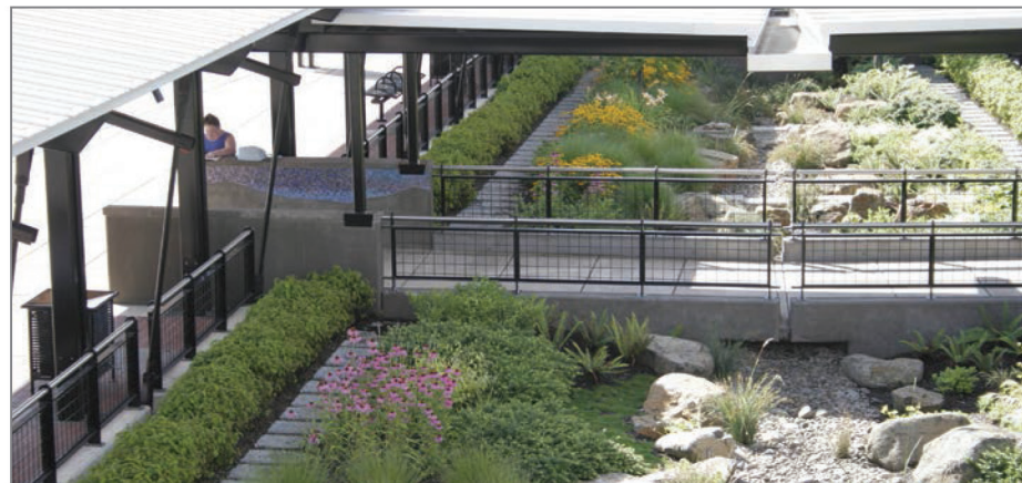
At Springfield Station, rain filters into a garden where it is cooled and treated.
