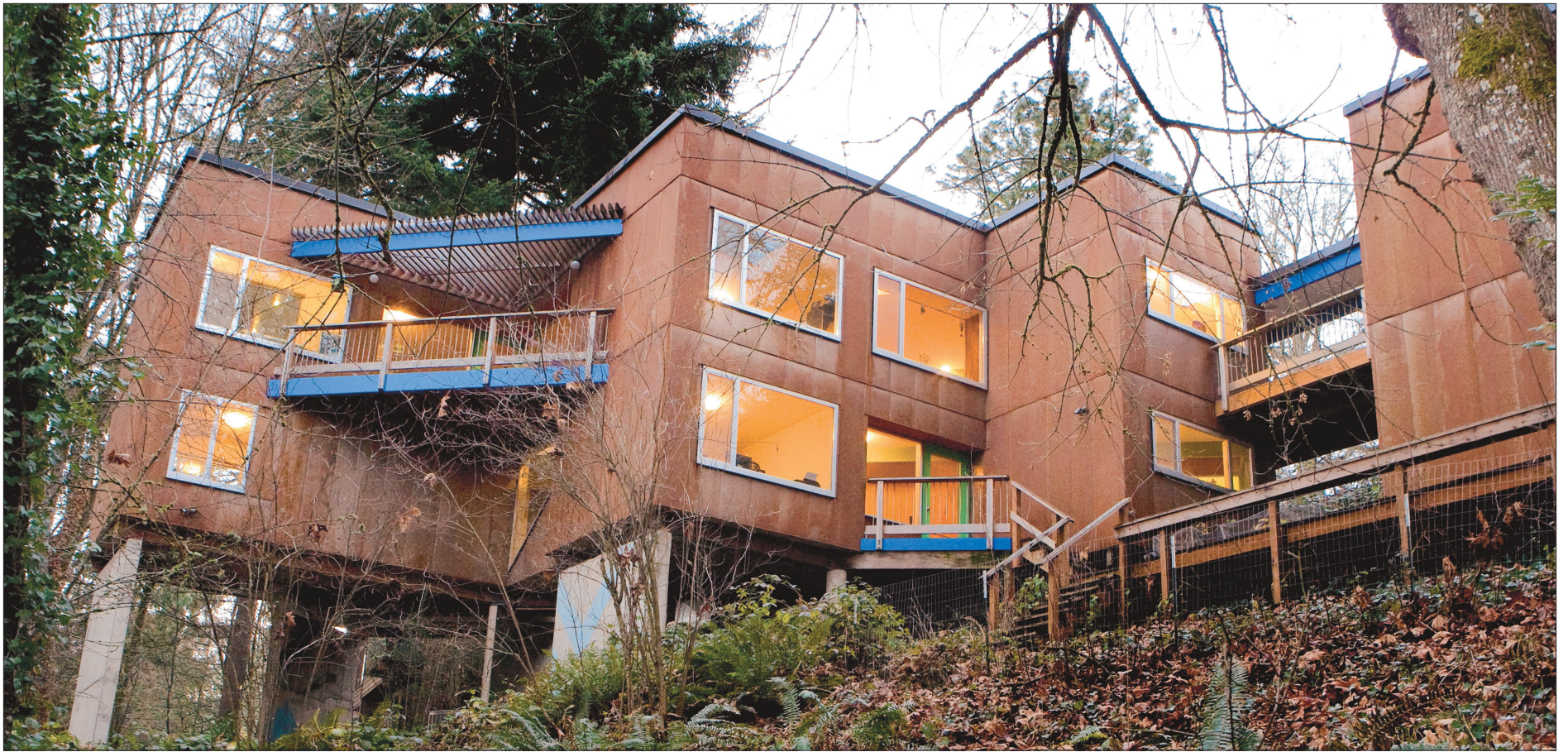
Blocks of living spaces rest on concrete walls to support 2,100-square-foot, late '60s home designed by former UO architecture professor and dean Robert Harris, now of Southern California.
