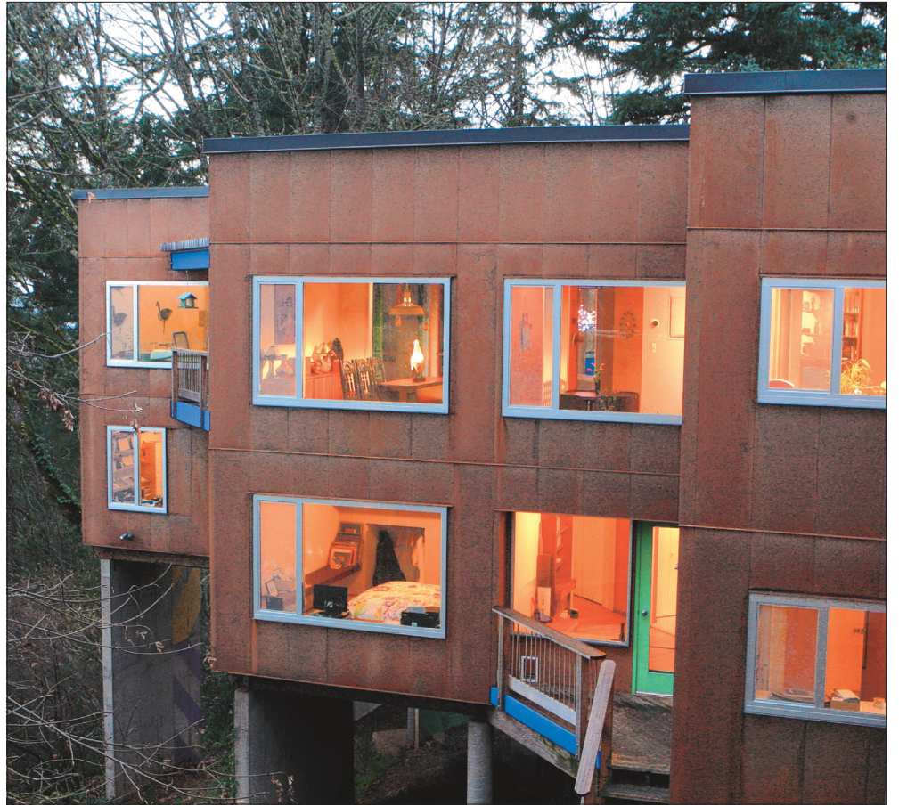
Corten steel now replaces the home's original redwood exterior siding.
