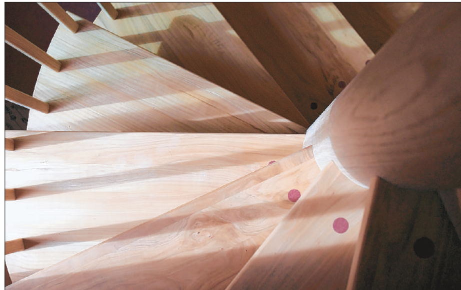
With an exacting fit, each riser looks like an organic extension of the center column on these stairs, which Kelly recently installed in an addition to a Eugene home.
